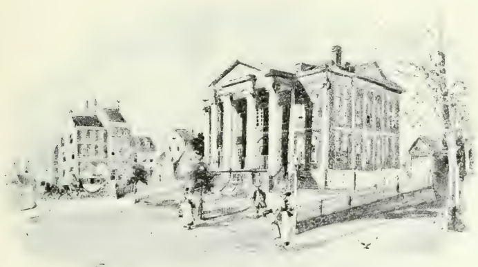
GOVERNMENT HOUSE AT THE BATTERY, NEW YORK, 1790
